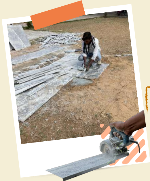
They measured the wall size and start cutting the granite ,and also made sides smooth
