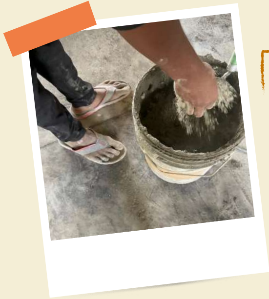
In my school construction was happening in the first floor
